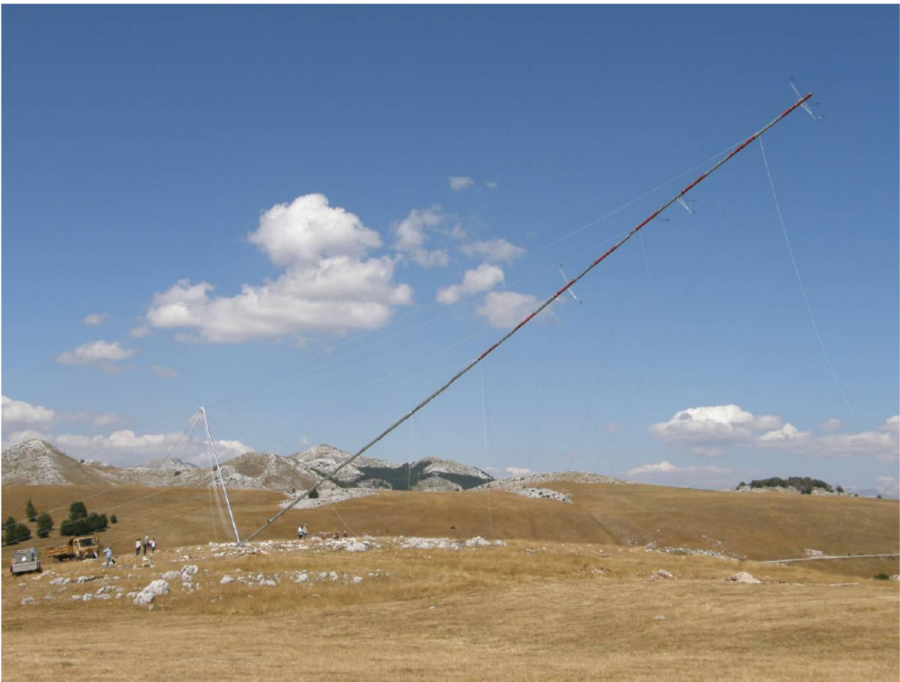
Installation of a measuring mast at Krnovo
